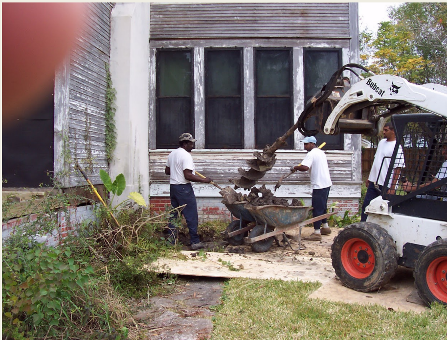
Chambers House Restoration Work Begins, 2004
