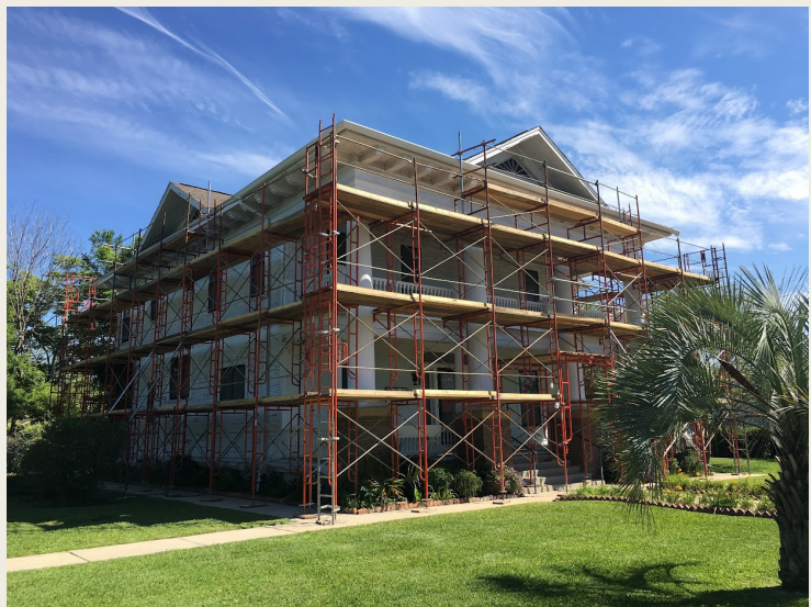
Chambers House under construction
